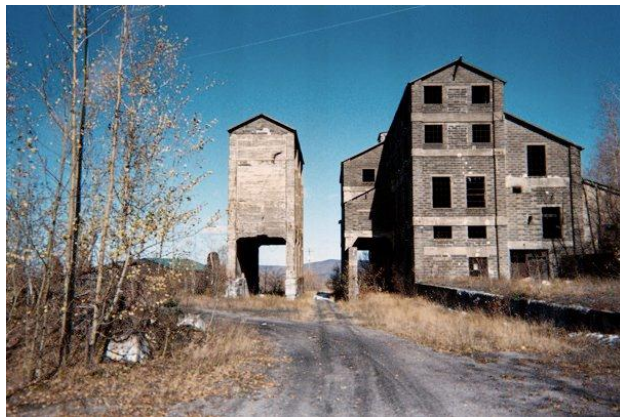
Fig 4: Loading facilities for hopper cars on railroad spur lines
